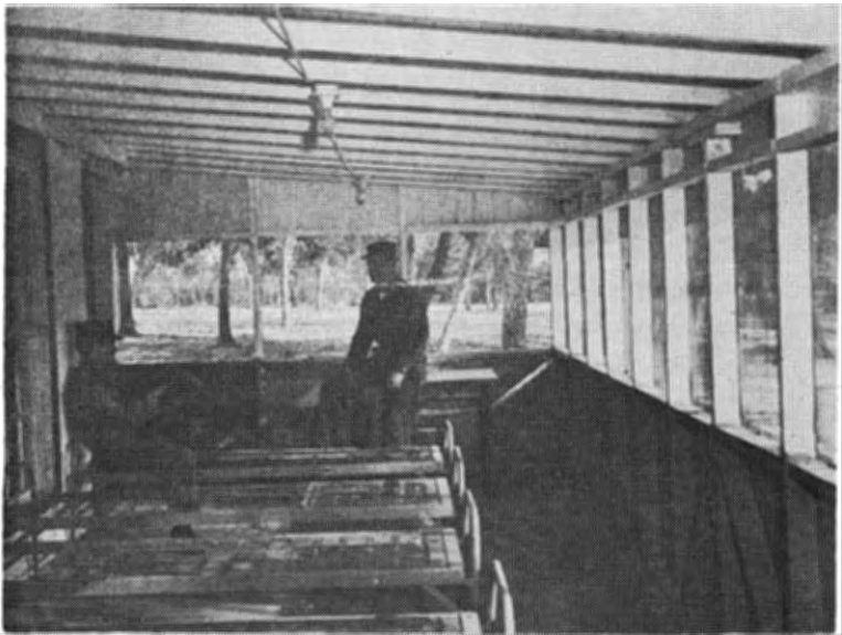
HERE IS SHOWN ONE OF THE COMPLETED OUTSIDE PORCHES ADDED TO EACH CABIN. AS SHOWN AT LEAST 7 ADDITIONAL BEDS CAN BE SET UP ON THIS PORCH, OR IT CAN BE USED FOR CARD PLAYING, EATING WHAT HAVE YOU. ELECTRICAL OUTLETS AND LIGHTS ARE AVAILABLE ON THE PORCH.
