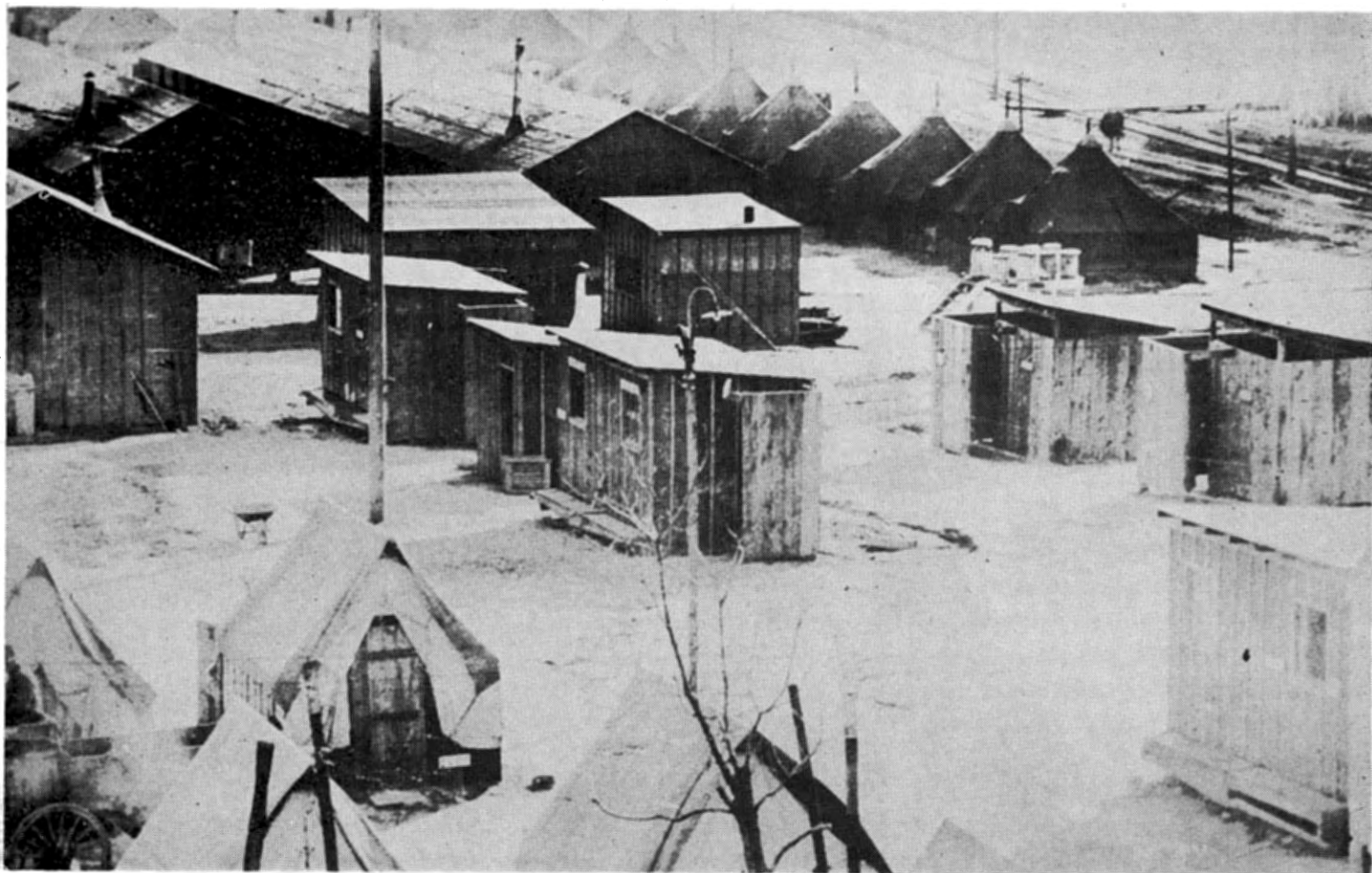
OUT OF A CARLOAD OF ASSORTED PIPE, A MILLION FEET OF LUMBER, AND THE EFFORTS OF 600 WORKMEN LABORING ON THE DOUBLE-QUICK FOR SEVEN DAYS, THE FIRST HOME OF THE PRESENT INFANTRY SCHOOL ROSE PROUDLY BUT UNLOVELY IN 1918 ON MACON ROAD, THREE MILES FROM COLUMBUS.
