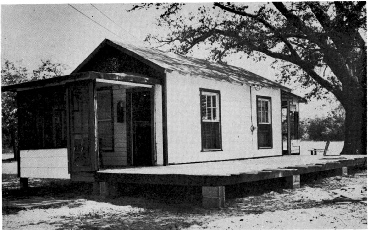
THIS SHOWS ONE OF THE CABINS PRIOR TO THE MAJOR UPLIFTING IT RECEIVED. AS SHOWN HERE, A LARGE SCREEN PORCH IS STARTING TO GO UP
