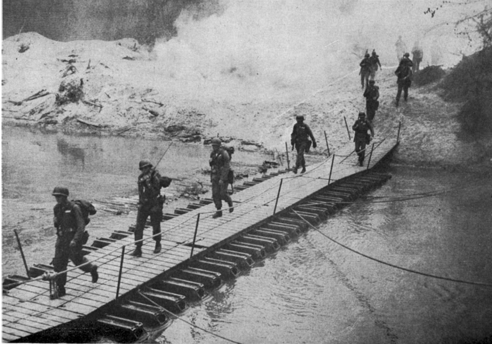
THE ORDER TO MOVE OUT UNDER COVER OF A SMOKE SCREEN IS GIVEN TO FOX COMPANY, 135TH INFANTRY REGIMENT. THE PONTOON BRIDGE WAS ERECTED BY THE 682ND ENGINEERS.
