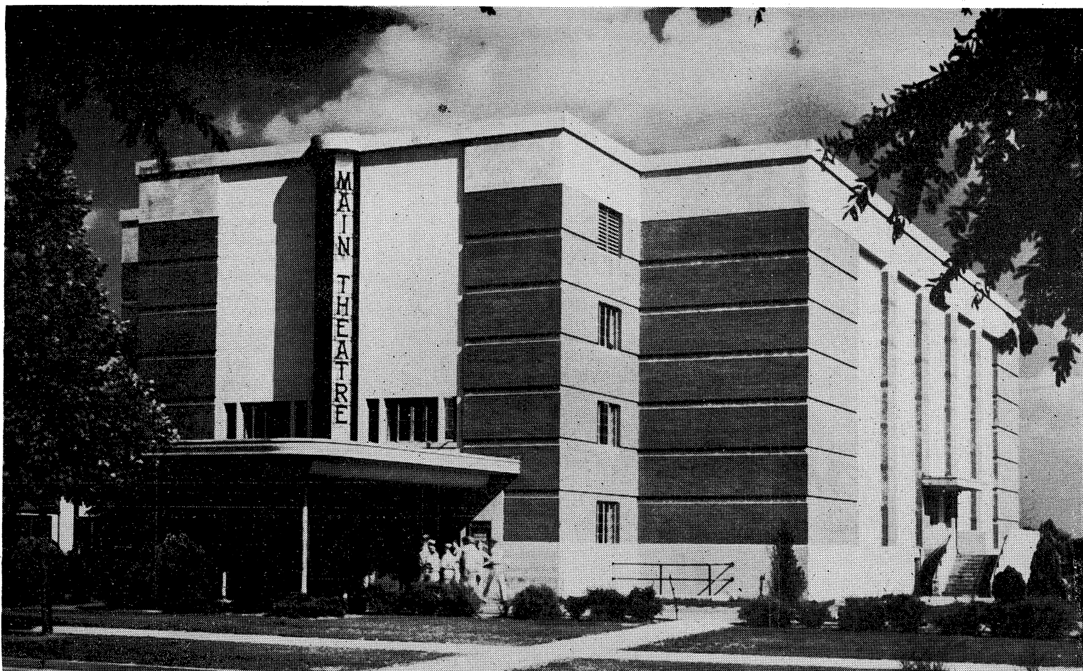
MAIN THEATER: BUILT IN 1938, THIS THEATER IS ONE OF THE LARGEST MILITARY THEATERS IN THE UNITED STATES. IT HAS A SEATING CAPACITY OF OVER 1,500 AND IS SAID TO HAVE THE FINEST ACOUSTICS OF ANY THEATER IN THE COUNTRY. THE ENTIRE BUILDING IS FULLY AIR CONDITIONED. THEATER ACTIVITIES, OTHER THAN MOVIES, INCLUDES GRADUATION EXERCISES, PRESENTATION OF NAME BANDS, PLAYS, CHORAL GROUPS AND ADDRESSES BY DISTINGUISHED VISITORS TO FORT BENNING. THERE ARE A NUMBER OF OTHER THEATERS, MOSTLY OF TEMPORARY CONSTRUCTION, LOCATED THROUGHOUT THE POST.
