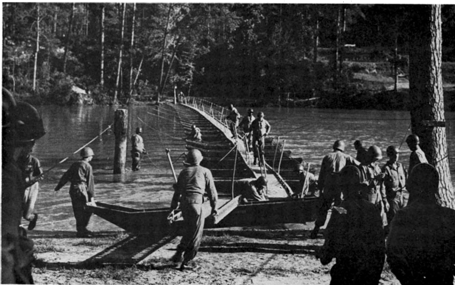
FOOT BRIDGES ACROSS SWIFTLY FLOWING STREAMS ARE CONSTRUCTED BY THE 78TH ENGINEERS.
